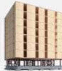
Timber 7 Timber Floors & Shear Walls; Steel Frame Podium
