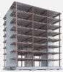
Ref 1 Concrete Slabs on Steel Deck; Steel Frame; Concrete Cores
