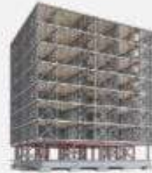
Timber 8 Timber Floors; LGM Framing; Steel Frame Podium
